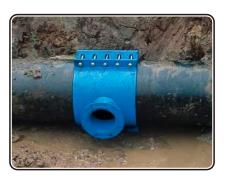
We also use engineering steel to make DN 200 - DN 1200 two-part split collars, flanged two-part split collars, adapters to connect different pipe sizes, and other untypical pipe fittings.
